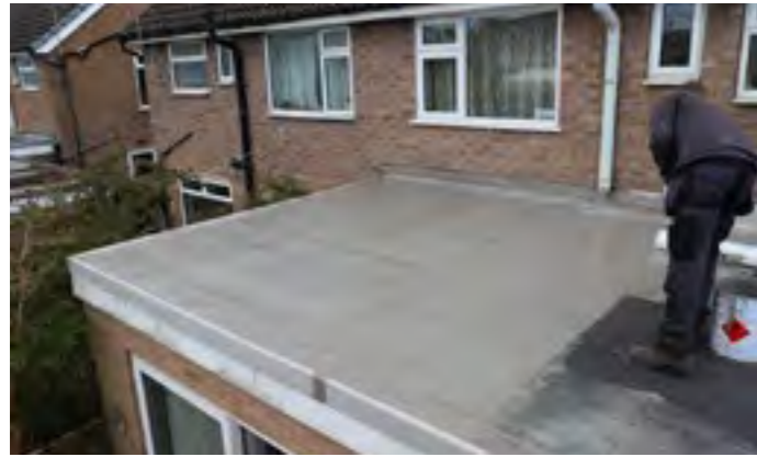
Two people are required for laminating the roof. One to apply the basecoat with a soft roller and another to consolidate with a paddle roller.
